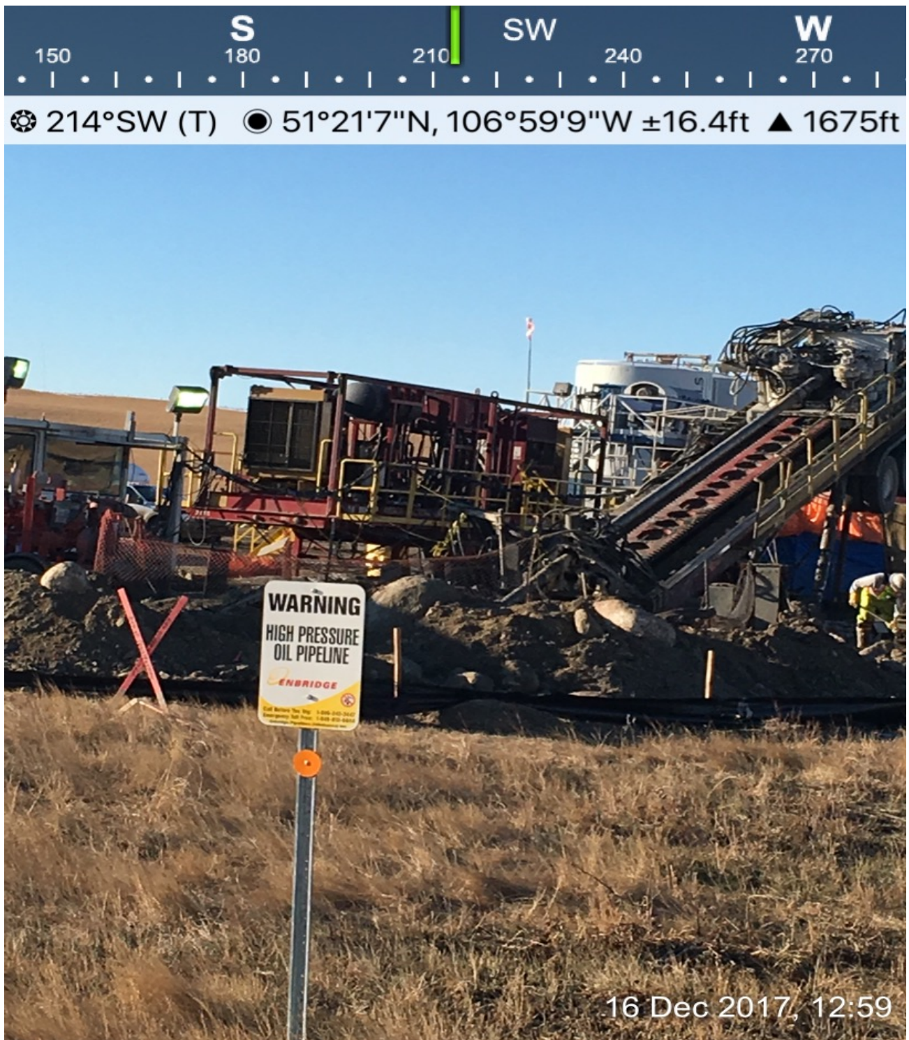
HORIZONTAL DIRECTIONAL DRILLING ENTRY POINT
