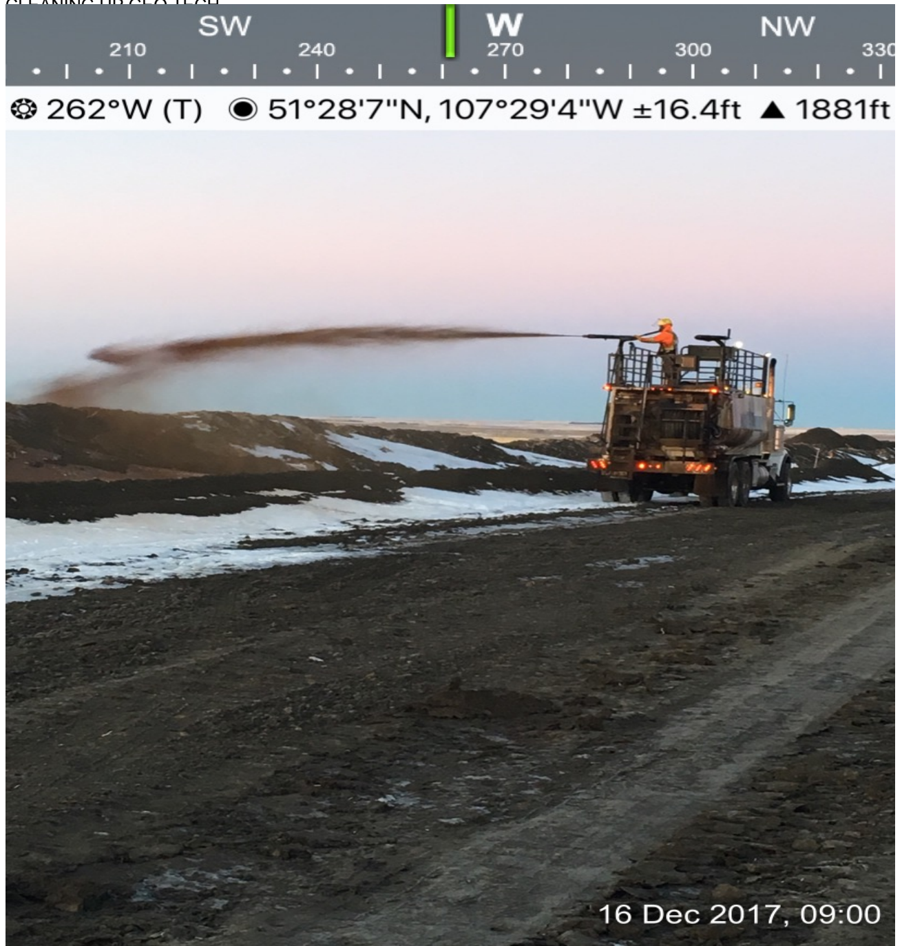
TACKIFYING SOIL ERROSION PREVENTION METHOD
