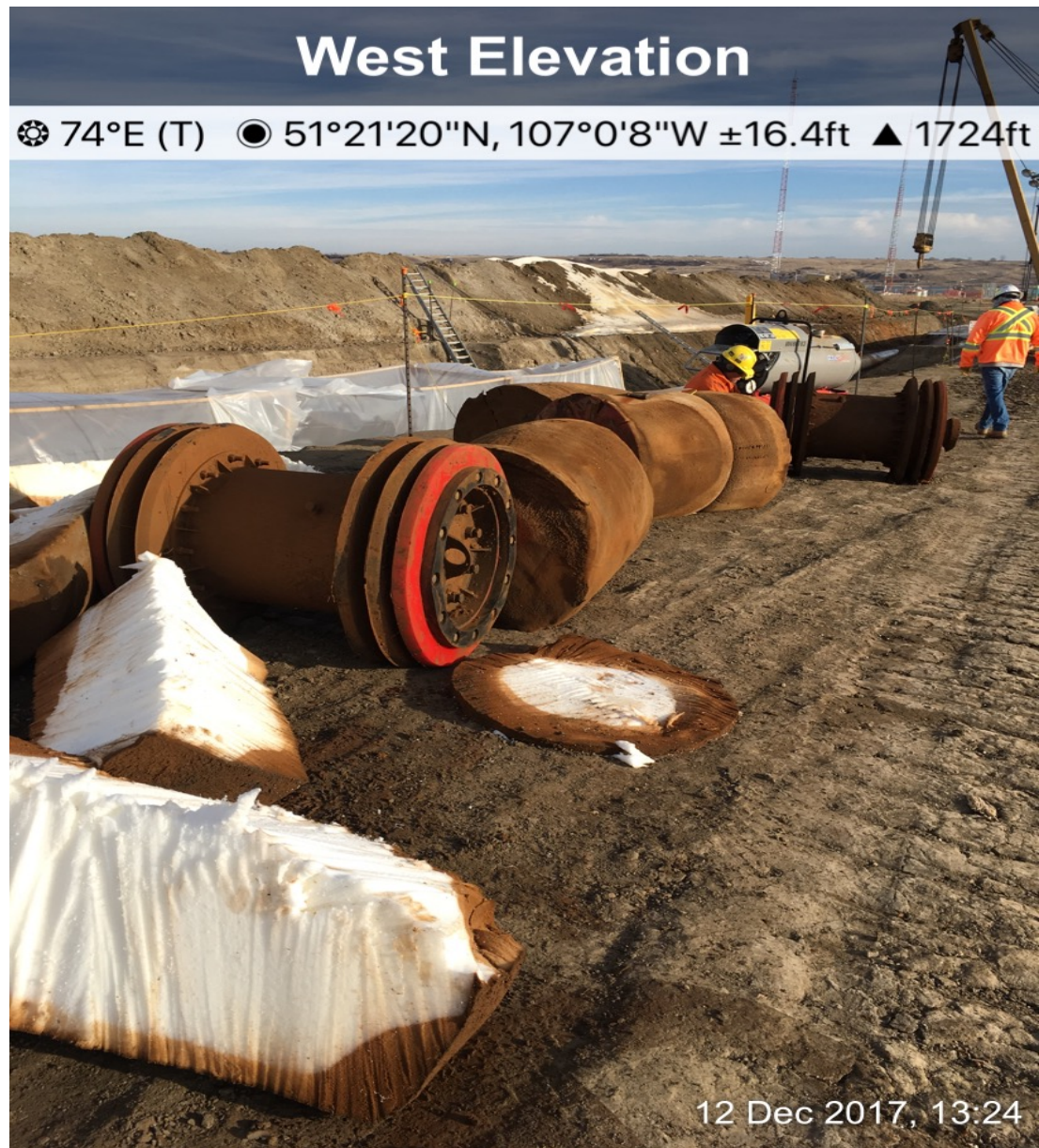
PIGS THAT CAME OUT OF THE MAINLINE AFTER HYDRO TEST
