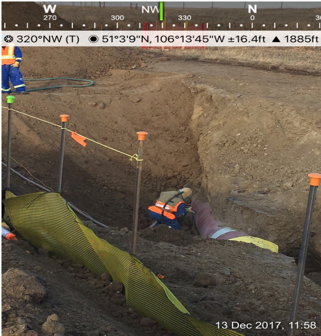
REPAIRING COATING
